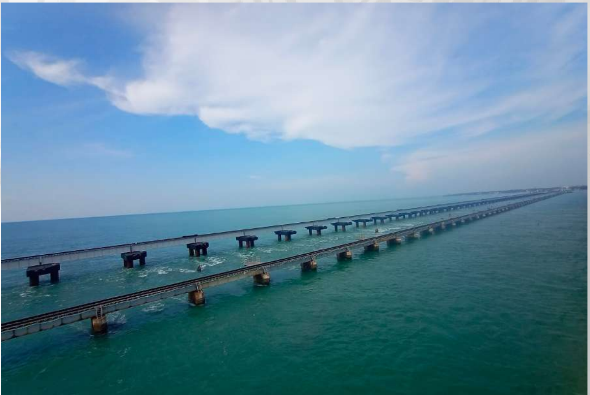
Hardik Poddar, Class 10 Photo Location: Pamban Bridge, Tamil Nadu Mobile Photography
